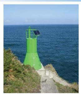
Mediterraneo's GRP towers, model MTP, are engineered to integrate flashing and rotating beacons c/w their solar power supply system, in order to operate as medium- and long-range Lighthouses.
